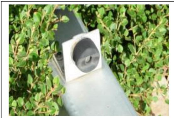
Ensure stops are installed on the gate for the fully closed and fully open positions.
